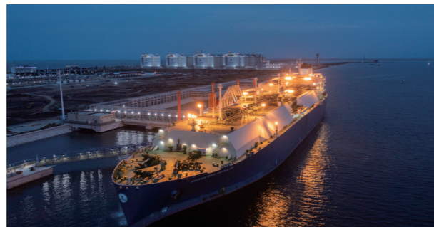
Customized measures for each vessel ensure safe and reliable LNG unloading
